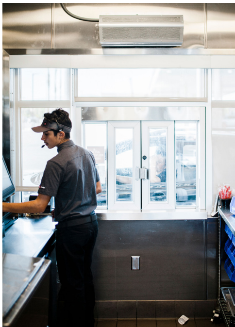
PASS-THRU WINDOW: The pass-thru window is protected from fumes, exterior (untreated) air, flying pests and keep workers much more comfortable.
