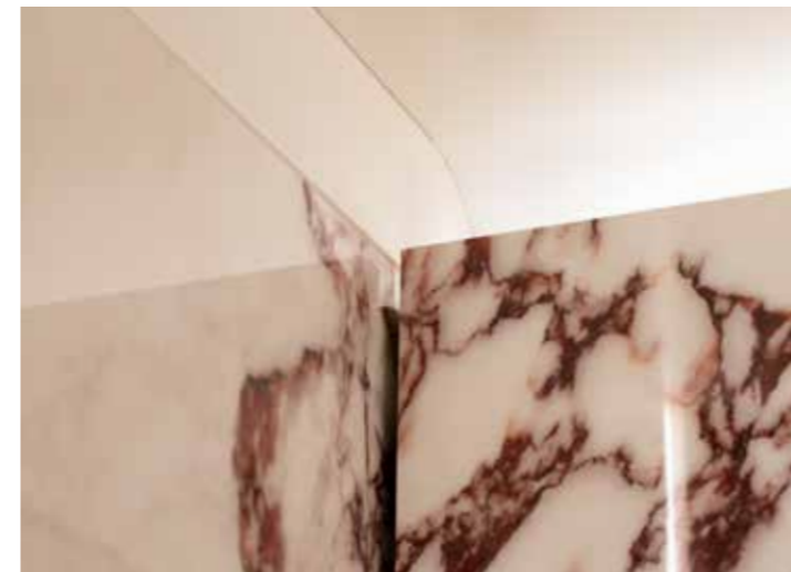
Viola rossé stoneware back and sides details; air supply from the top of the back panel
