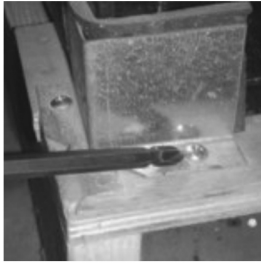
Image 1 Removing bracket from skid
