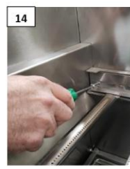
BURNER CONNECTING SHEET SCREWS ARE INSTALLED
