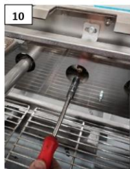
REPLACED INJECTOR IS FITTED
